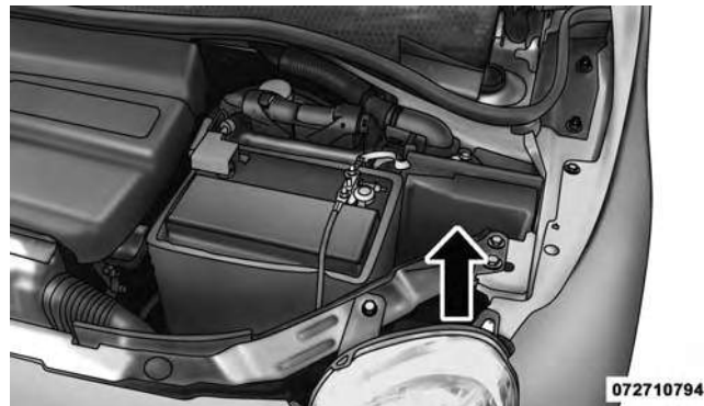
Front Distribution Unit
